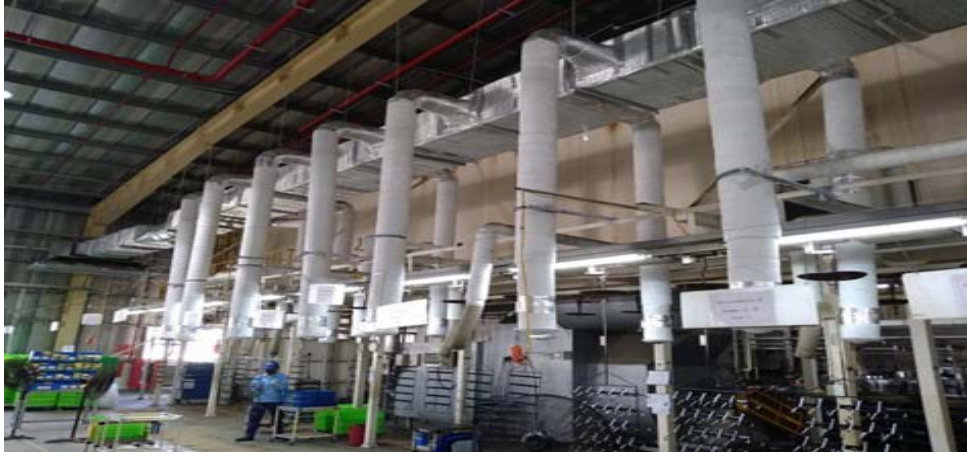
<Sprinkler pump equipment>
